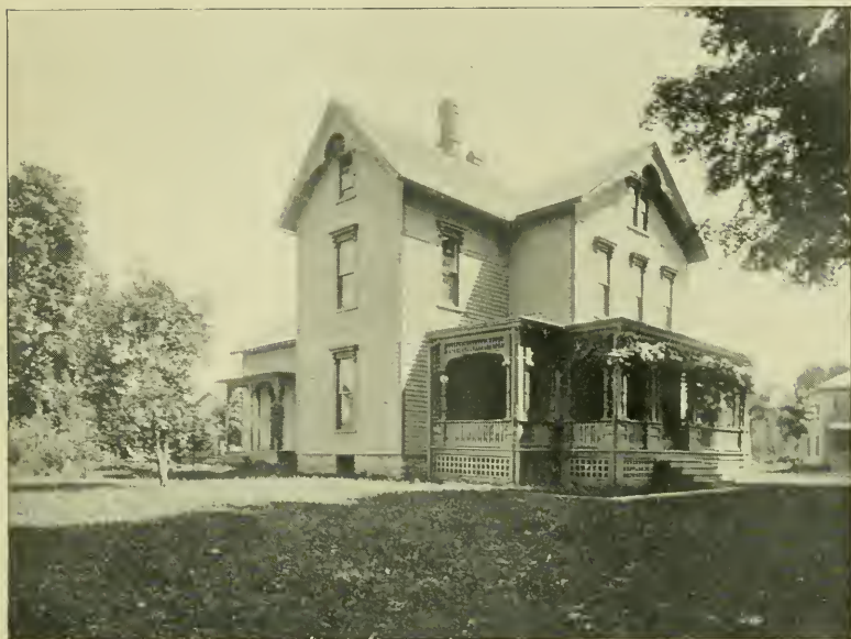
RESIDENCE OF A. C. STAFFORD, JAMESTOWN STREET.
