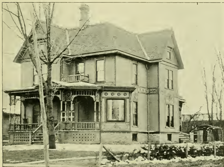
RESIDENCE OF J. A. BESTRUP, ERIE AVENUE.
