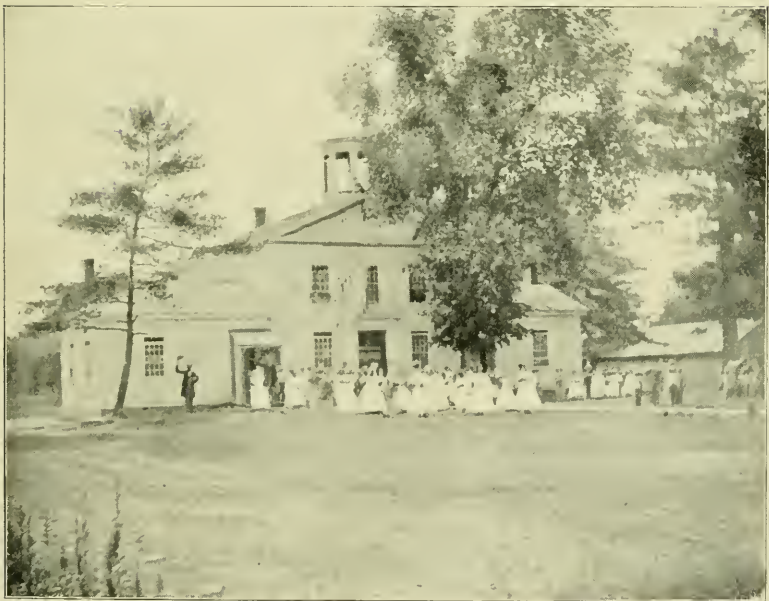
GOWANDA UNION SCHOOL. BUILT, 1844. BURNED, AUGUST 9, 1874.
